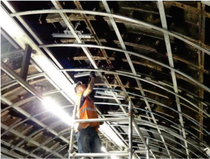
Unistrut bracket installation at Vauxhall station
