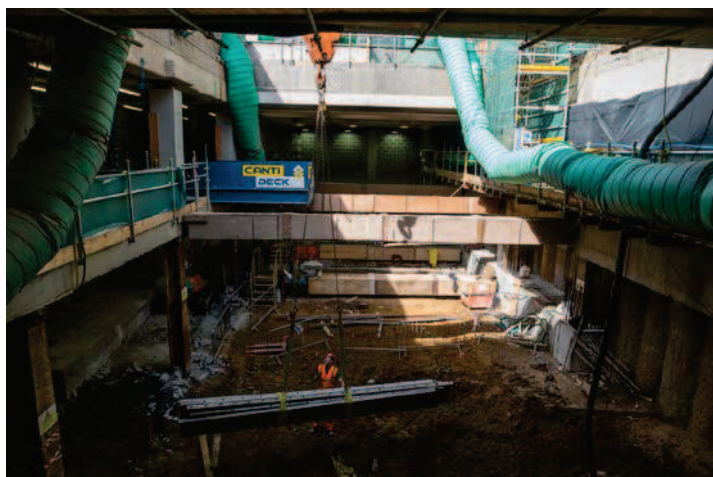
Victoria station north ticketing hall lifting operations
