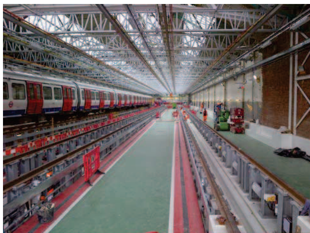
S-Stock train in the upgraded Ealing Common depot shed
