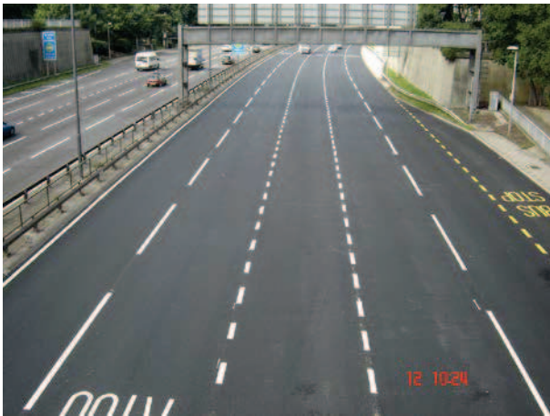
A406 five lanes Eastbound at High Road Bridge
