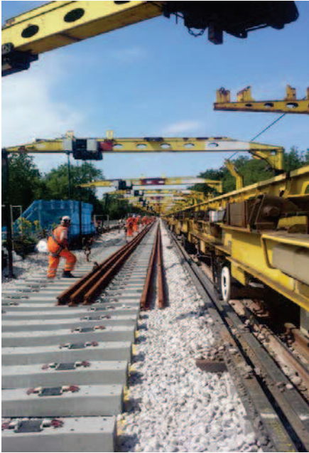
New rails at a site near Ickenham during Uxbridge block closure
