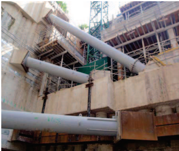
Temporary propping of the LU box at Bank station
