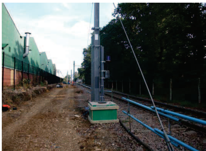
Twin tracking works
