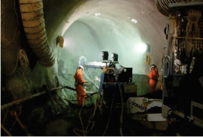
Bond Street station shaft | excavation works
