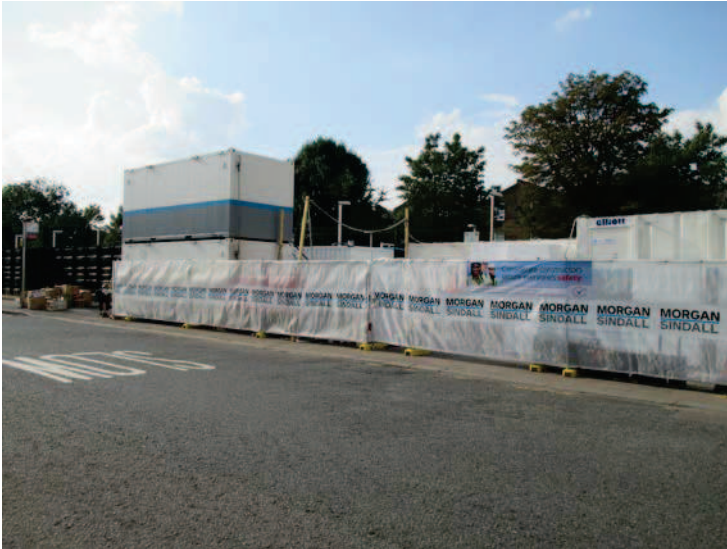
Kensal Rise station site set up
