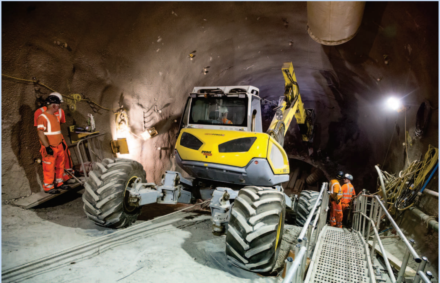
Victoria station upgrade, showing excavation below existing concourse
