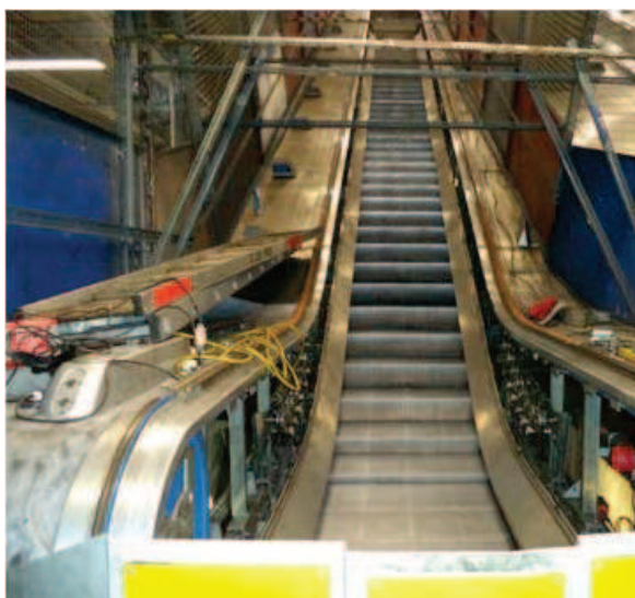
Canada Water escalator installation
